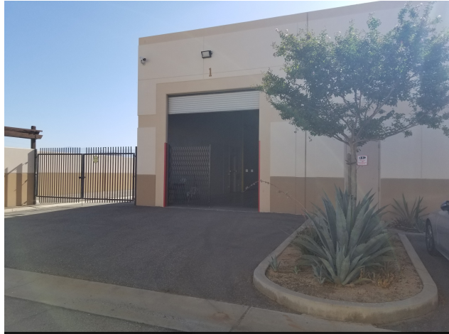
Ground Level Door
