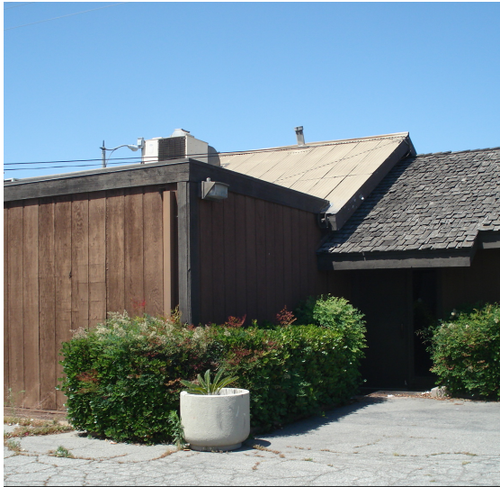
View of Office Building
