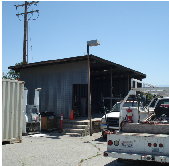
Covered Storage Building
